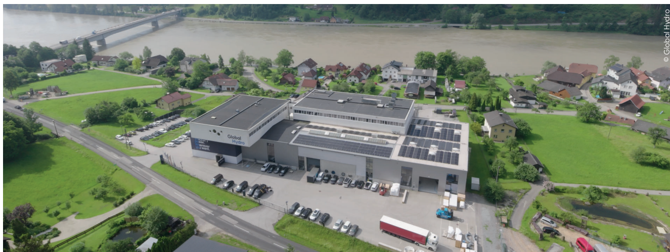
As with various other digital solutions, Global Hydro is an industry pioneer in hydropower service field development.
