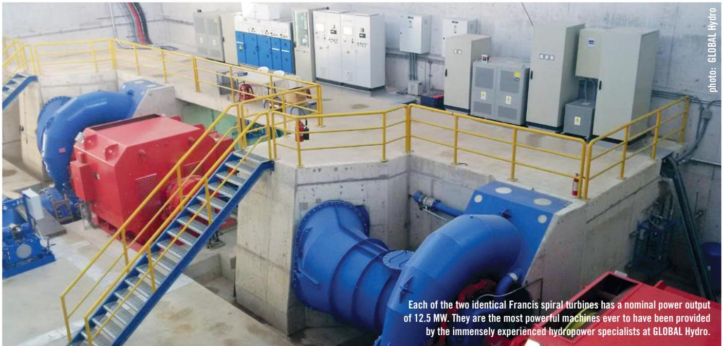
Each of the two identical Francis spiral turbines has a nominal power output of 12.5 MW. They are the most powerful machines ever to have been provided by the immensely experienced hydropower specialists at GLOBAL Hydro.
