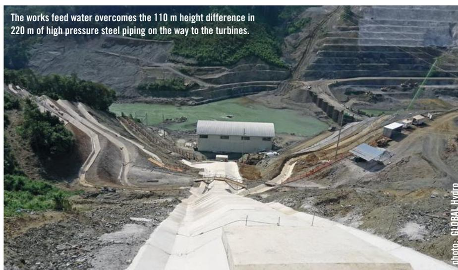
The works feed water overcomes the 110 m height difference in 220 m of high pressure steel piping on the way to the turbines.
